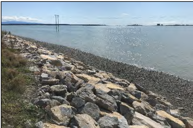
Rip rap seawall, southeast estuary
