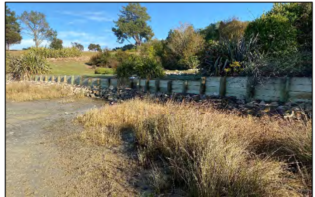
Seawall, Hoddy arm
