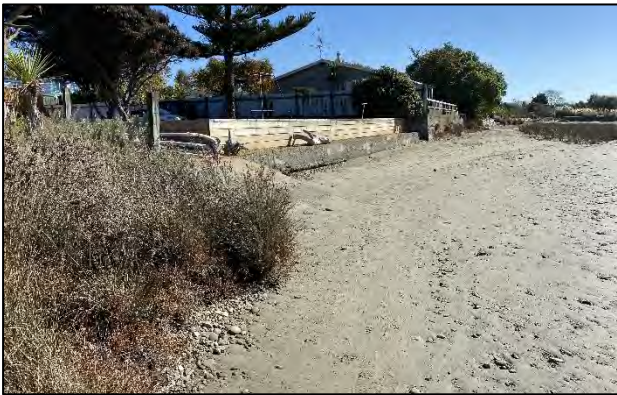
Small area of saltmarsh and residential seawalls in Mapua
