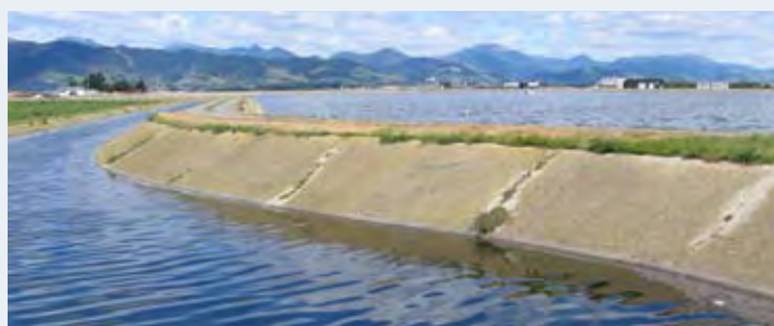
Bells Island Regional Sewage Authority point source discharge of treated wastewater to Waimea Inlet.
