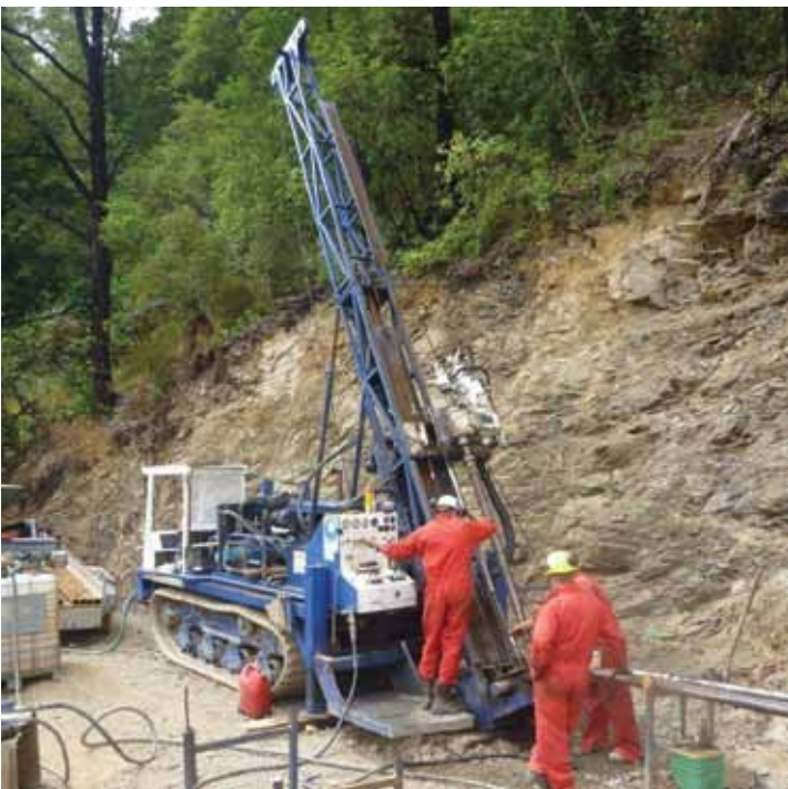
Clockwise L-R: Core samples of the dam foundation rock; drill rig crosses the Lee River near the dam site; drillers near the dam site record water flow; drillers make a drill hole at an angle on the right abutment of the river.
