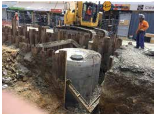
Figure 2: flood mitigation works in Queen street - Richmond
