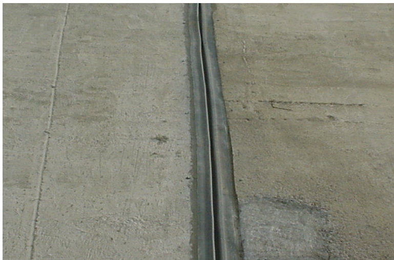
Figure 7-9 External Omega Seal
