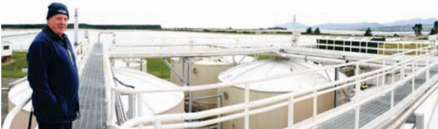
Nelson Regional Sewerage Business Unit facilities at Bells Island.
