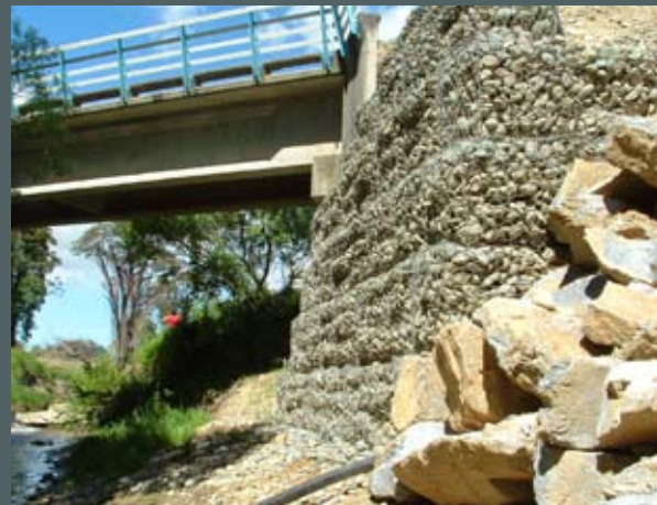
Sherry Road Bridge.
