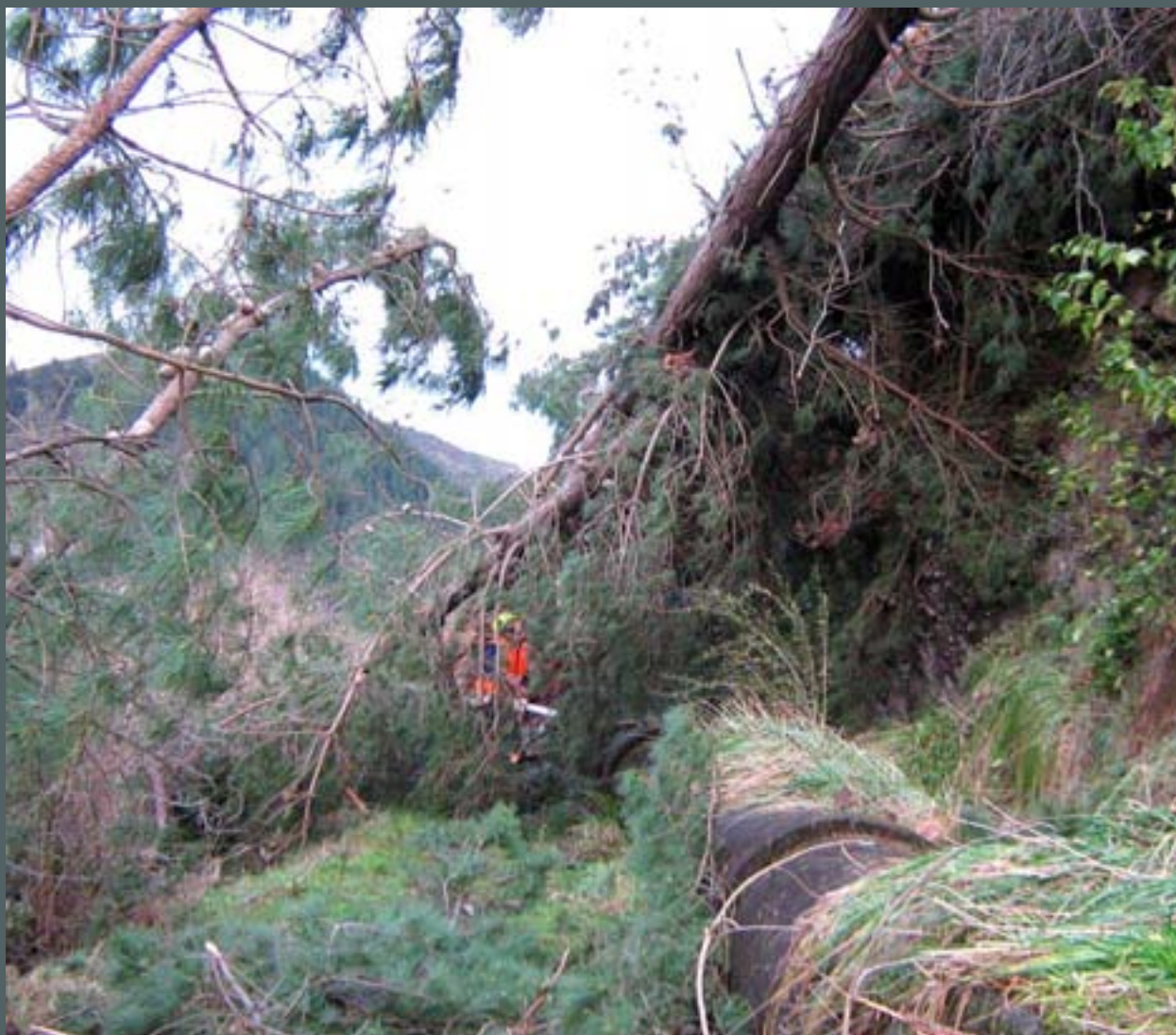
Repairing the Maitai pipeline.
