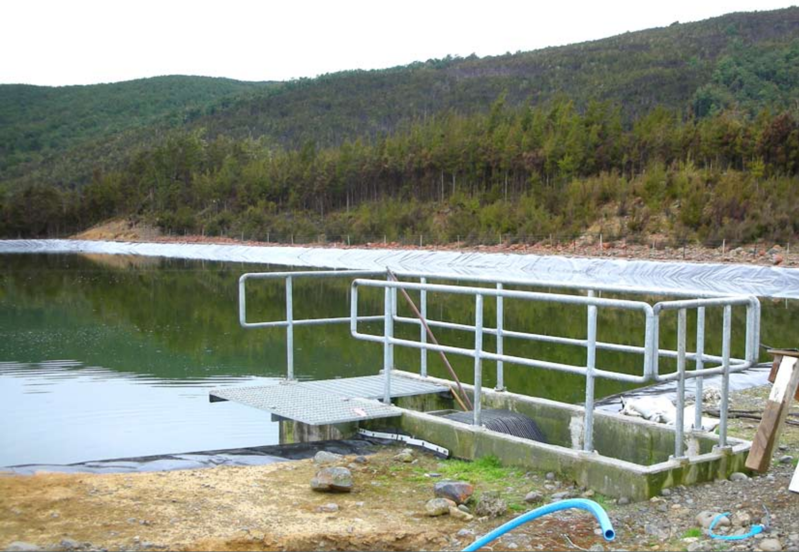
St Arnaud wastewater treatment plant.
