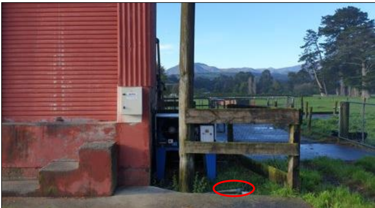
Figure 3: Bore located in low lying area. Runoff from the milking shed is likely to soak into the ground near the bore.
