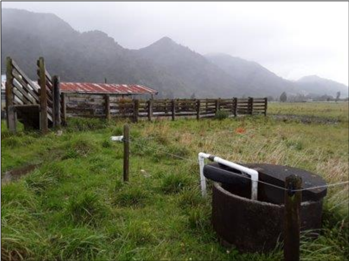
Figure 4: Well located in paddock without an adequate well head protection. Contamination can easily enter into the groundwater from the well.
