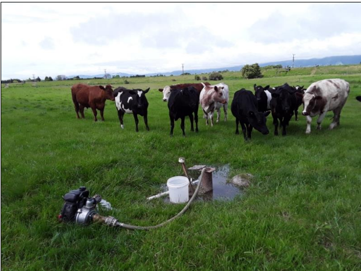
Figure 5: Bore located in paddock with no fencing to prevent stock from accessing the bore. Though the riser is above the ground surface, the bore itself is located in a low-lying area where water tends to pool with no concrete pad to prevent soakage. Contamination is likely to soak into the ground near the bore or have floodwaters flow directly down the bore.
