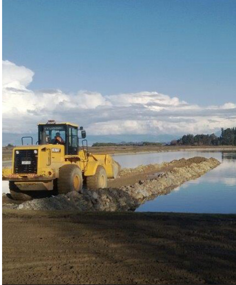
Bund construction at Motueka's wastewater plant
