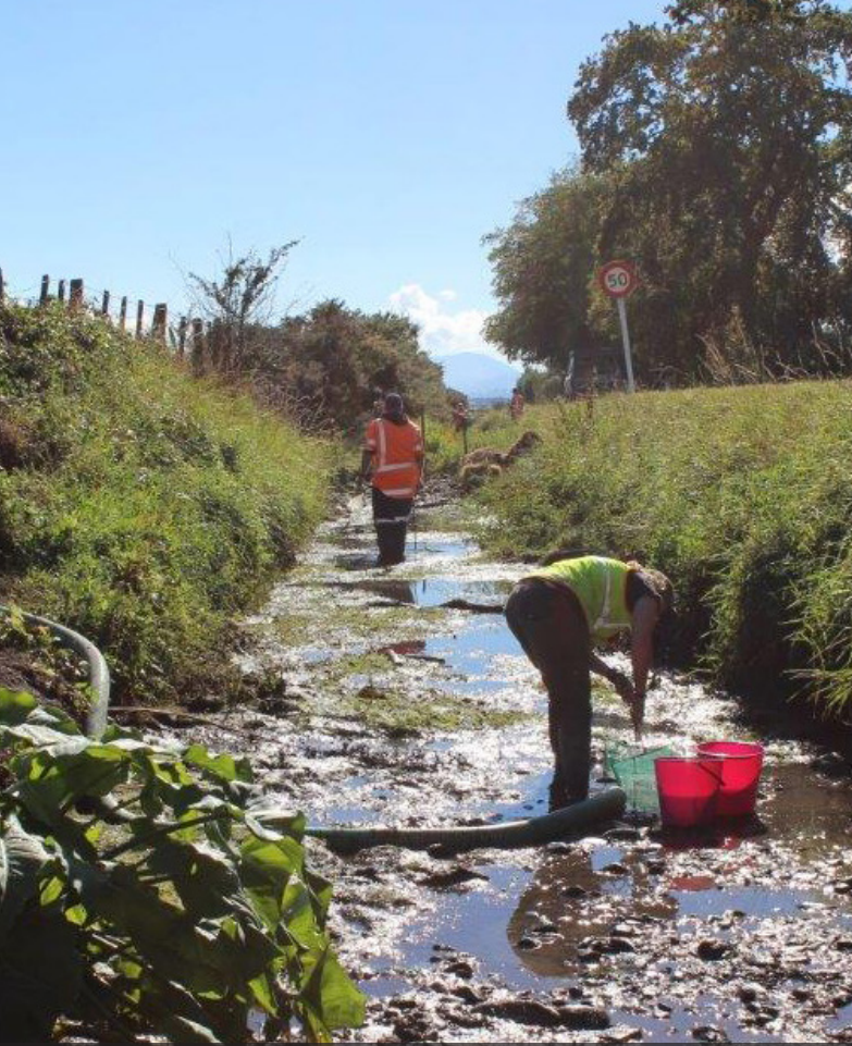
Supporting Richmond stormwater capacity upgrades: Borck Creek
