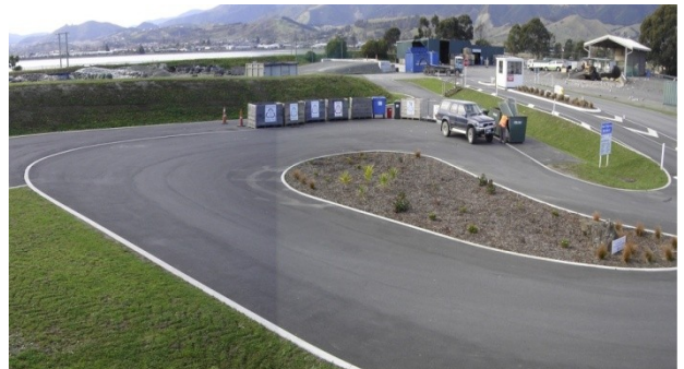
Richmond Resource Recovery Centre upgrade
