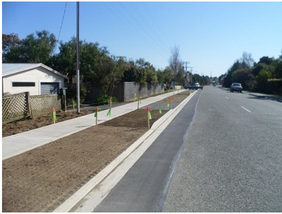
Aranui Road upgrade
