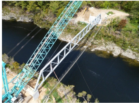
Reconstruction of James Road Bridge in Golden Bay
