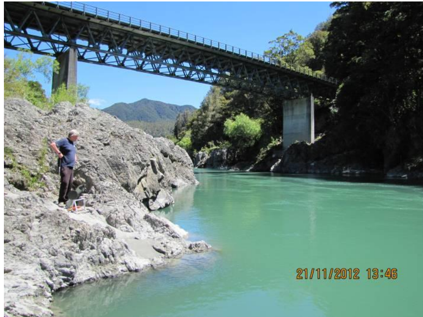
Above: Buller River upstream O’Sullivan Bridge (SH6) (November 2012)
