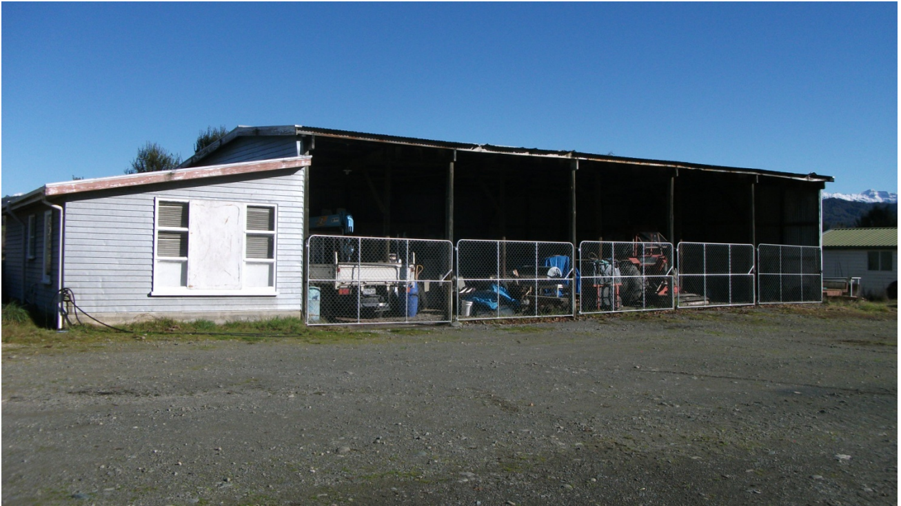
Old works depot Tapawera
