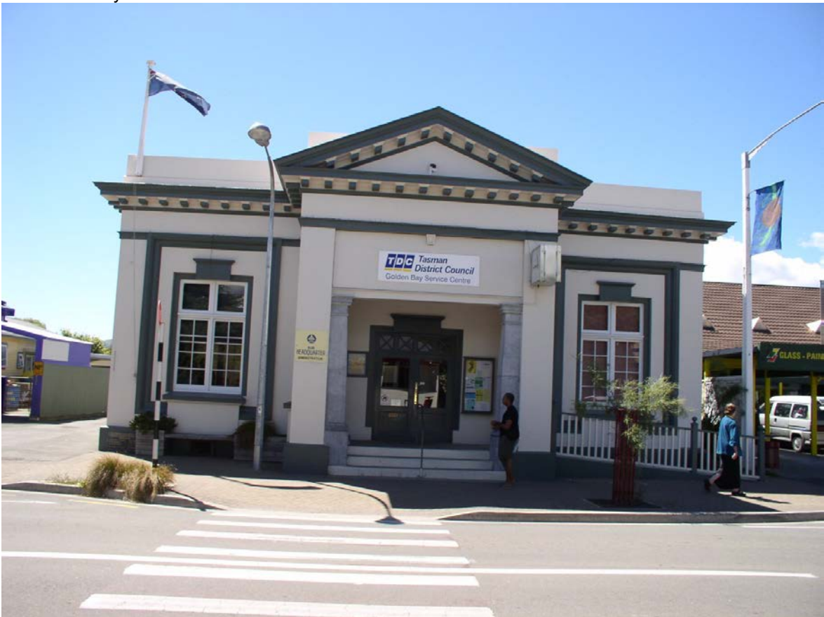
Golden Bay Service Centre taken 2009 – Closed pending Seismic repairs.
