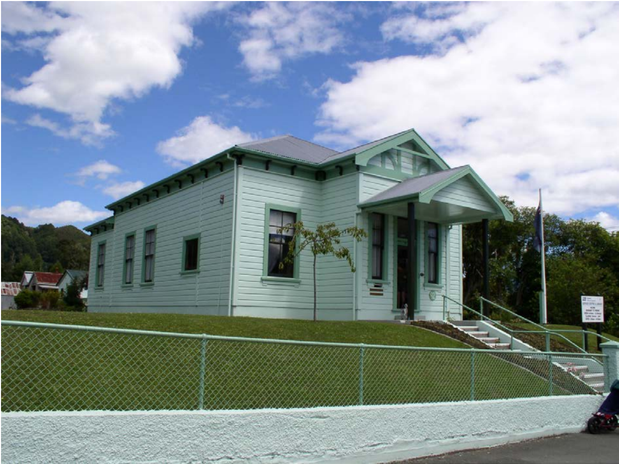
Murchison Service Centre and Library
