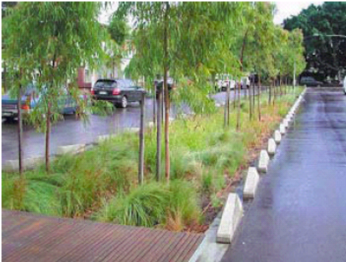
Figure C3a Rain garden in a residential street
