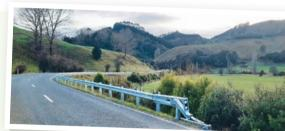
The Tasman Alliance and specialist supply partner JC Contracting installed a 384m guardrail on steel-driven posts. The finished result is functional, looks good, and will no doubt stop more vehicles from falling off the side of this stretch of road.
