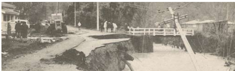
The Brook Stream turned into a raging torrent.
