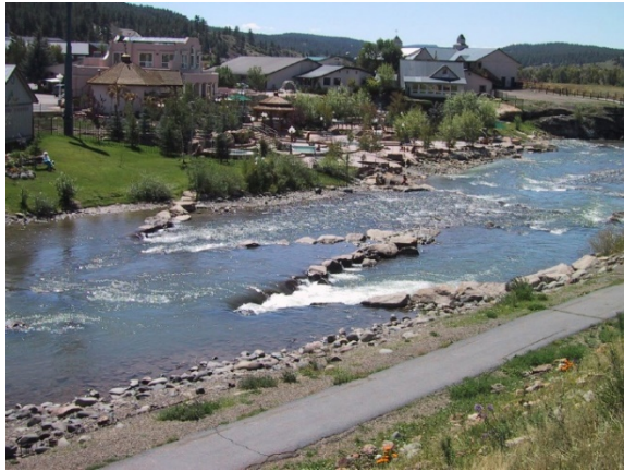
Example of a W-rock weir in a large river in America (Conejos Canyon Ranch, 2001).
