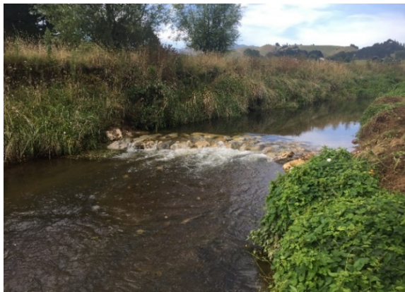
An example of a simple rock weir in a Waikato Stream, note the variety of rock sizes (WRC unpublished).
