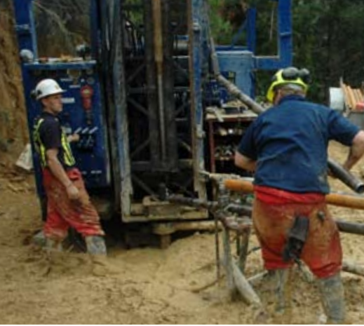
Drillers collecting rock core samples. Waterfall Flat, which is part of the dam footprint.
