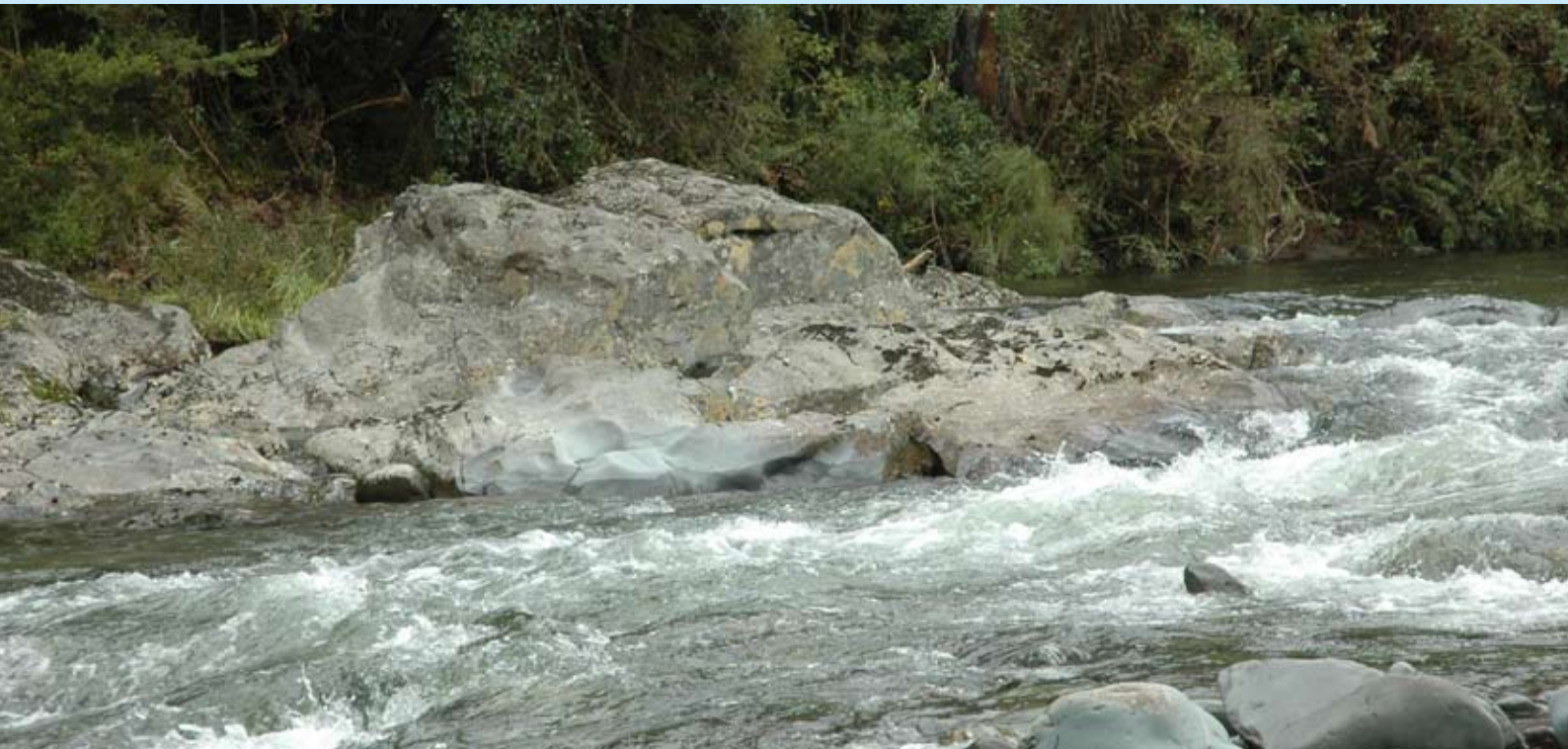
Possible upstream dam site in the Lee River.
