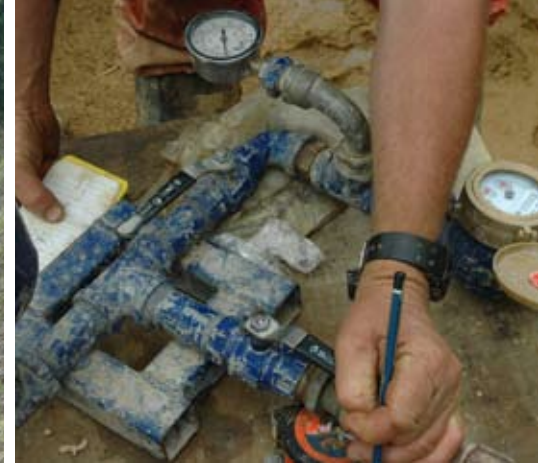
Pressure testing one of the sample bores.
