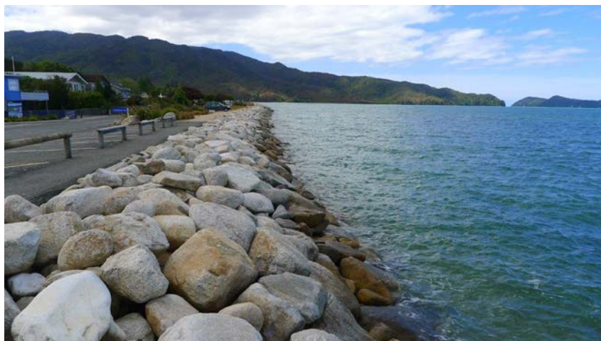
Figure B-2: Marahau Sea Wall
