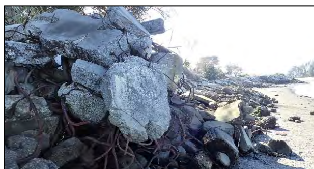
Steep-faced rock seawall in the northwest estuary
