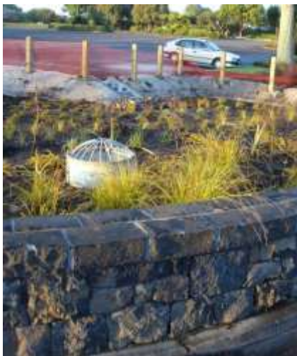
Raingarden treating parking lot runoff shortly after planting, showing the overflow, and after about three years; a diverse range of native groundcovers is used including coprosmas, shrubby pohuehue, sedges and Astelia, with lancewood providing interest.
