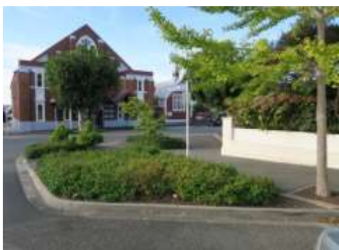
Bioretention can be located to provide multiple benefits: these three locations protect pedestrians from traffic, maintain clear views of intersections by preventing parking, and also receive the dirtiest runoff (corners are where brakes and tyres are worn, and spills are most likely to occur). Left – bump out in Nelson city could be converted to a raingarden; centre – bump out raingarden protects a bus stop and pedestrian crossing (Portland, Oregon, before planting); right – turn around raingarden with edges protected by boulders (North Harbour residential development).
