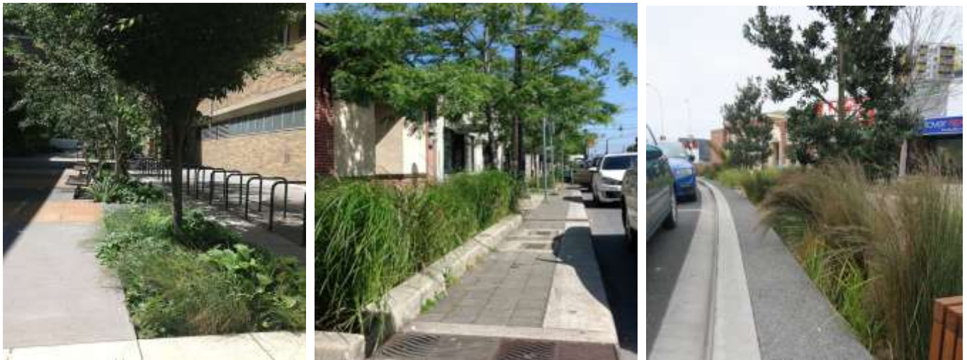
Effective placement of bioretention. Left – bioretention in a public through fare separates cycle parking from pedestrians ; Centre and right – bioretention set back from the road edge allows people to get out of cars and reduces need for traffic controls when trimming vegetation / removing litter (Portland, Oregon and New Lynn Auckland)
