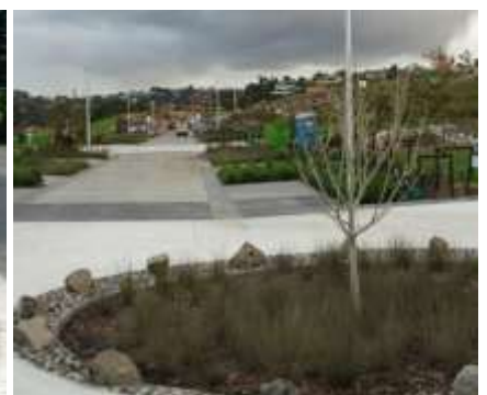
Bioretention can be located to provide multiple benefits: these three locations protect pedestrians from traffic, maintain clear views of intersections by preventing parking, and also receive the dirtiest runoff (corners are where brakes and tyres are worn, and spills are most likely to occur). Left – bump out in Nelson city could be converted to a raingarden; centre – bump out raingarden protects a bus stop and pedestrian crossing (Portland, Oregon, before planting); right – turn around raingarden with edges protected by boulders (North Harbour residential development).
