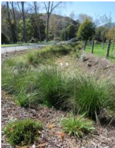
Nelson/Tasman Bioswale plantings. Left – stakes are used to allow fast identification for efficient weed control during establishment of this swale. Centre – a low-maintenance edge of gravel-mulched, short turutu ( Dianella nigra ) and taller oioi and knobby clubrush ( Ficinia nodosa ) in the centre. Right – Cyperus ustulatus in the centre of this raingarden is considered 'messy' by some people and may require removal of seed-heads to achieve suitable aesthetic outcomes in some localities.
