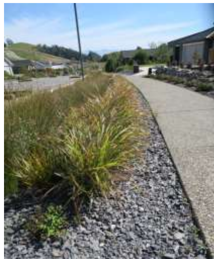
Nelson/Tasman Bioswale plantings. Left – stakes are used to allow fast identification for efficient weed control during establishment of this swale. Centre – a low-maintenance edge of gravel-mulched, short turutu ( Dianella nigra ) and taller oioi and knobby clubrush ( Ficinia nodosa ) in the centre. Right – Cyperus ustulatus in the centre of this raingarden is considered 'messy' by some people and may require removal of seed-heads to achieve suitable aesthetic outcomes in some localities.
