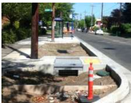
Bioretention can be located to provide multiple benefits: these three locations protect pedestrians from traffic, maintain clear views of intersections by preventing parking, and also receive the dirtiest runoff (corners are where brakes and tyres are worn, and spills are most likely to occur). Left – bump out in Nelson city could be converted to a raingarden; centre – bump out raingarden protects a bus stop and pedestrian crossing (Portland, Oregon, before planting); right – turn around raingarden with edges protected by boulders (North Harbour residential development).
