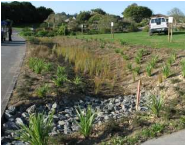
Bioretention swale about six months after planting and after about three years; plants on the well-drained edges are prostrate Coprosmas, prostrate manuka, mountain flax and scrambling pohuehue, with oioi in the wet base of the swale.
