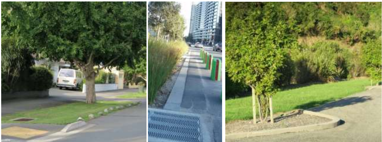
In the absence of a vertical 50 to 100 mm drop into a swale, physical barriers are usually important to exclude vehicles. Left – boulders used (Nelson); centre – bollards used (Melbourne); right – a clever use of curbs around trees (Nelson)
