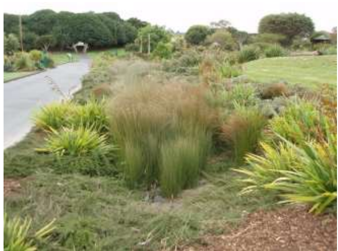
Bioretention swale about six months after planting and after about three years; plants on the well-drained edges are prostrate Coprosmas, prostrate manuka, mountain flax and scrambling pohuehue, with oioi in the wet base of the swale.
