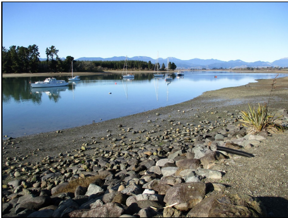
Figure 3: View looking south of the foreshore, in the approximate area of the planned boat ramp. Existing erosion protection in the foreground comprises large boulders tapering down to a muddy-sandy beach with loose gravel and boulders. The image was taken on 6 July 2022.
