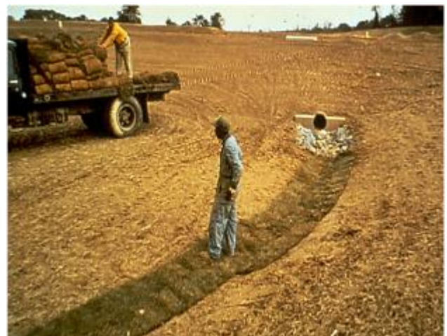
Figure 8-3326 Turf being applied for a swale outfall
