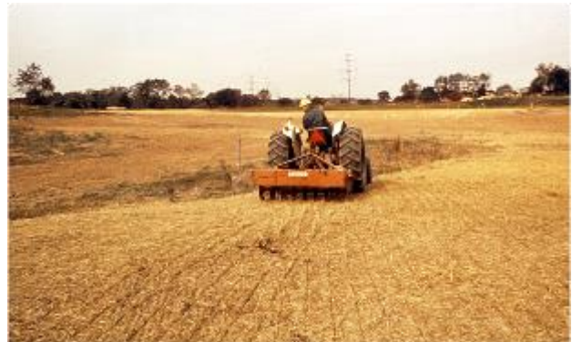
Figure 8-30 Straw mulch being crimped into ground to reduce windblown potential
