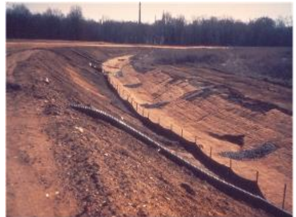
Figure 8-12 Pipe drop structure (note check dams, silt fence and channel protection also)
