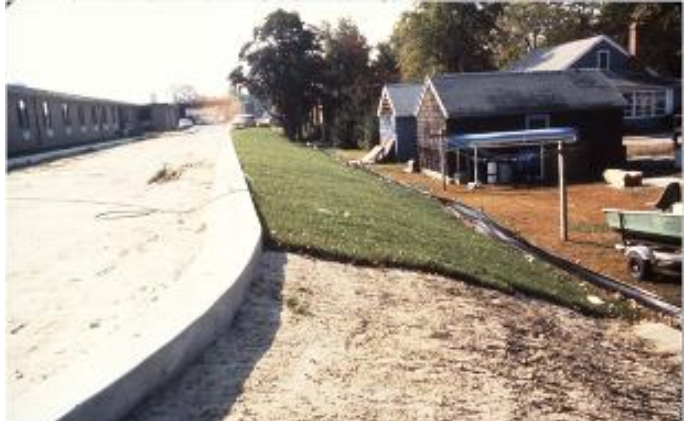
Figure 8-32 Turf being applied to provide immediate ground cover
