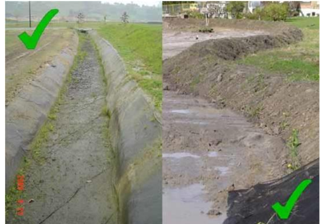
Figure 8-8 Diversions for intercepting clean water (left) and dirty runoff (Photos courtesy of BOPRC and Ridley Dunphy Environmental Limited)
