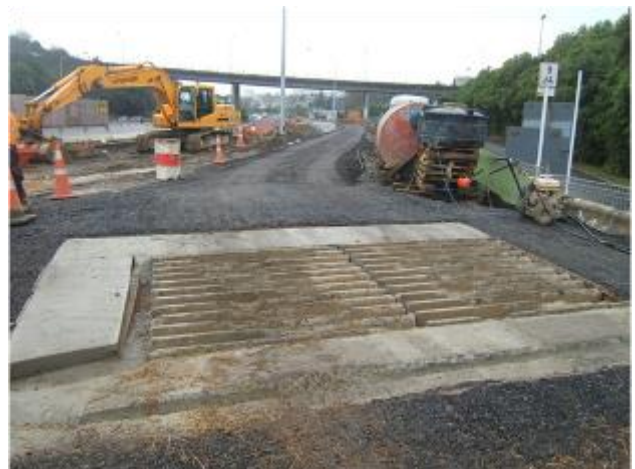
Figure 8-18 Example of a shaker ramp in site access point
