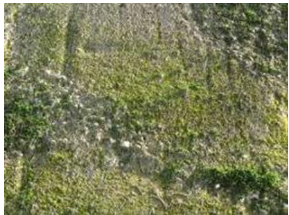
Figure 8-247 Recently applied hydroseed showing emergent grass growth
