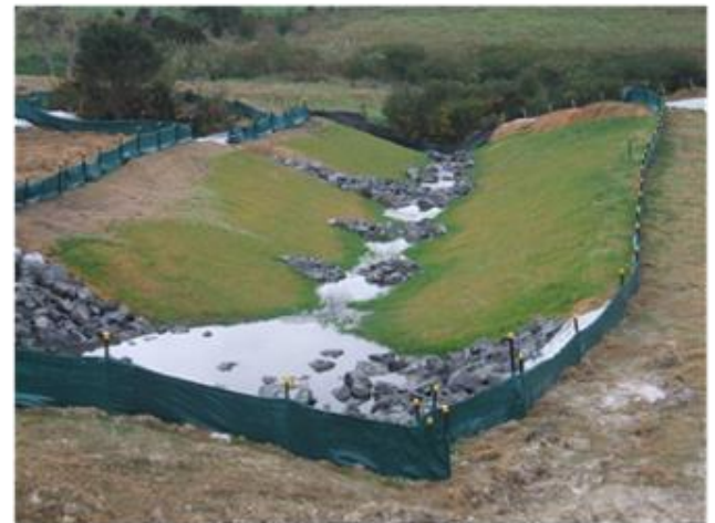
Figure 8-1 Check dams installed in series to act as a water velocity control measure
