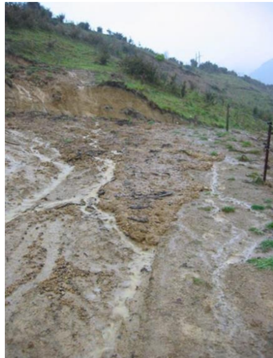
Figure 3-11 Mass Slumping in McConnon Creek Catchment
