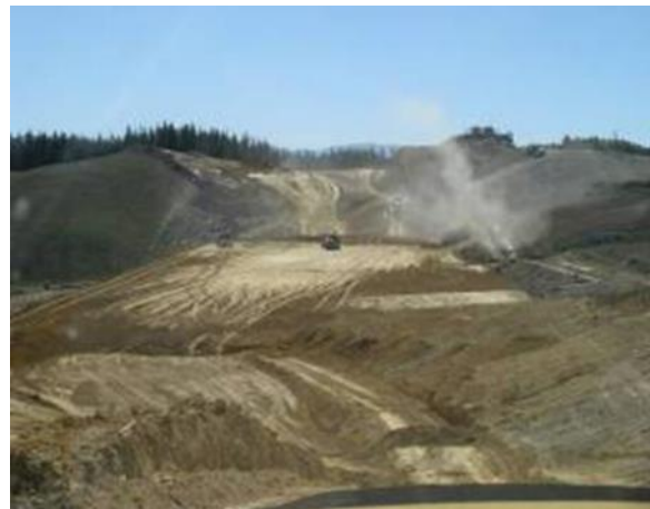
Figure 3-12 Wind Erosion on Ruby Bay Bypass
