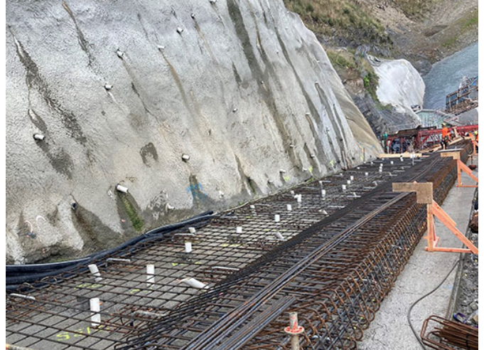
Figure 16: Steel fixing progress on RH plinth
