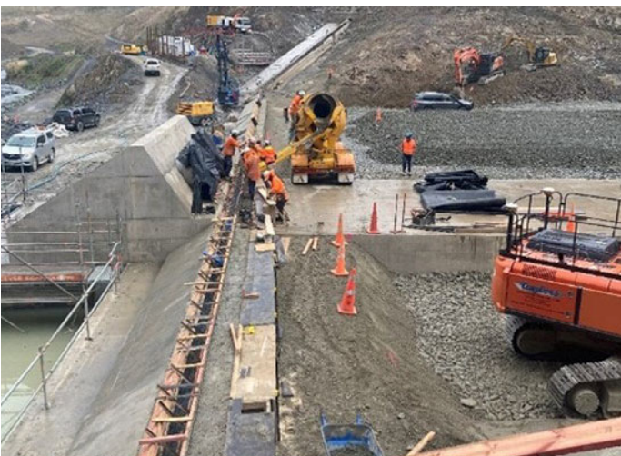
Figure 13: The first hand-made kerb is being placed
