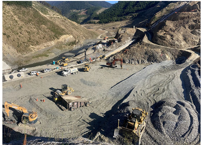
Figure 10: Upstream third embankment filling progress
