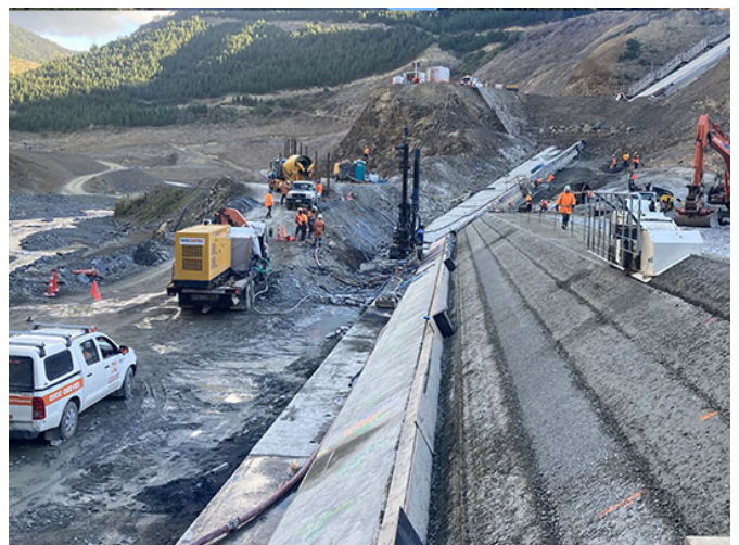
Figure 14: LH abutment foundation treatment & kerb placement
