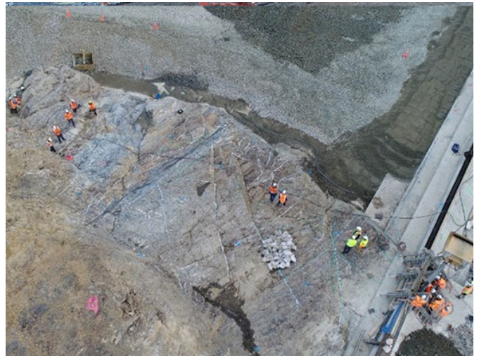
Figure 12: Cleaning LH abutment foundation
