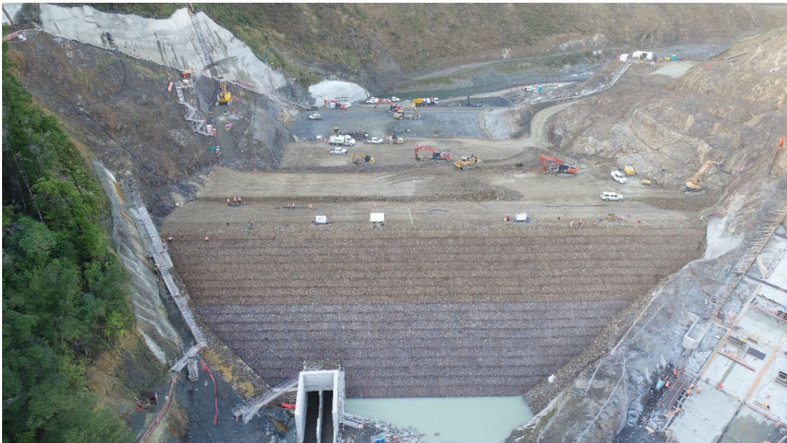
Figure 1: Reinforced Rockfill embankment viewed from downstream. Culvert on the left-hand side and spillway on the right of photo.
