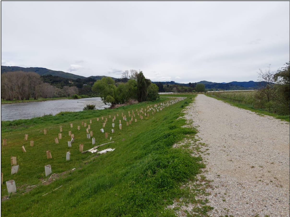
Figure 2: Planting of the floodplain as part of Whakarewa Street stopbank improvements
