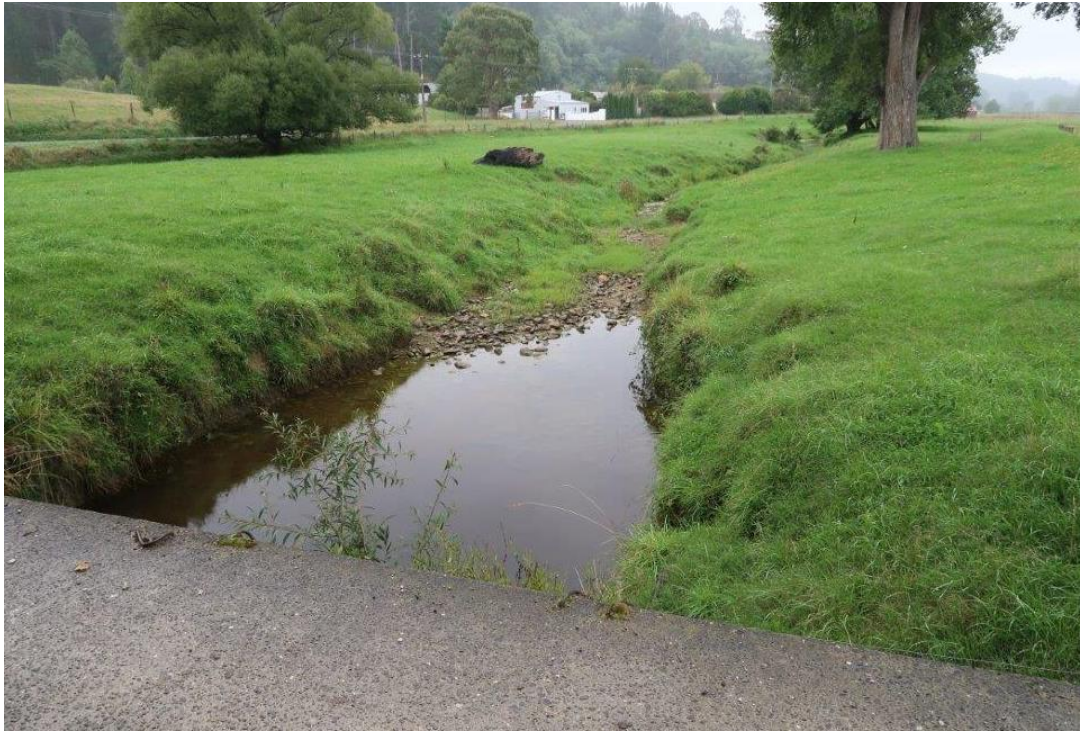
Fig. 4 Peach Island overflow channel immediately downstream of bridge. Dry sections of channel evident.
