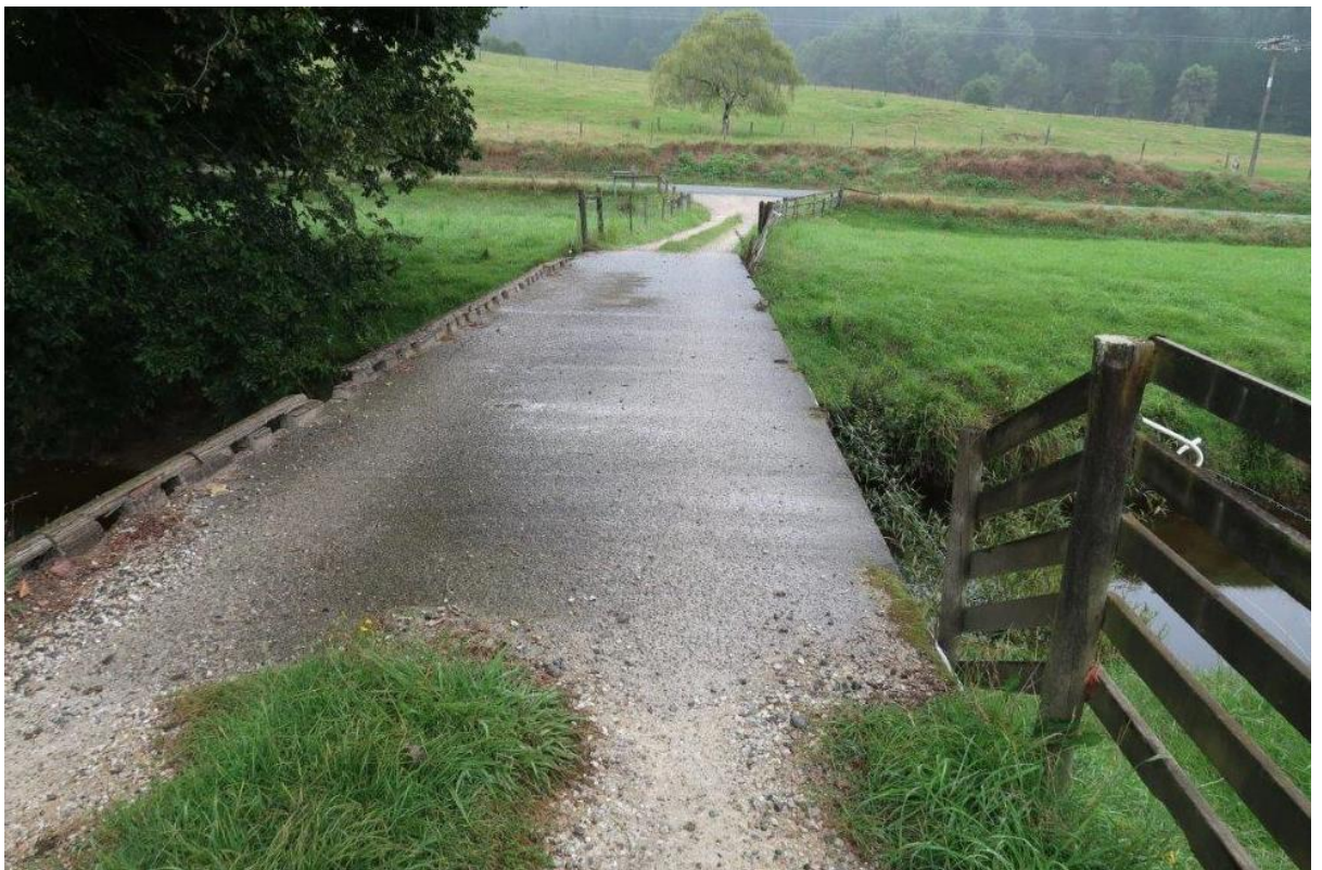
Fig. 3 Bridge over Peach Island overflow channel.
