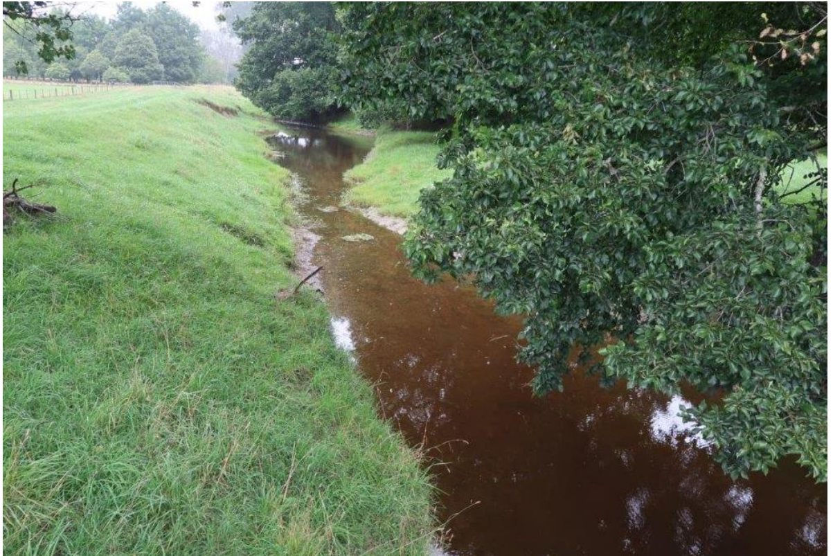
Fig. 2 Peach Island overflow channel immediately upstream of bridge.
