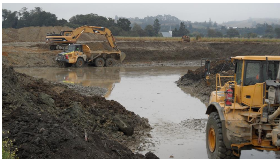
Figure 14. Excavation and backfilling.
