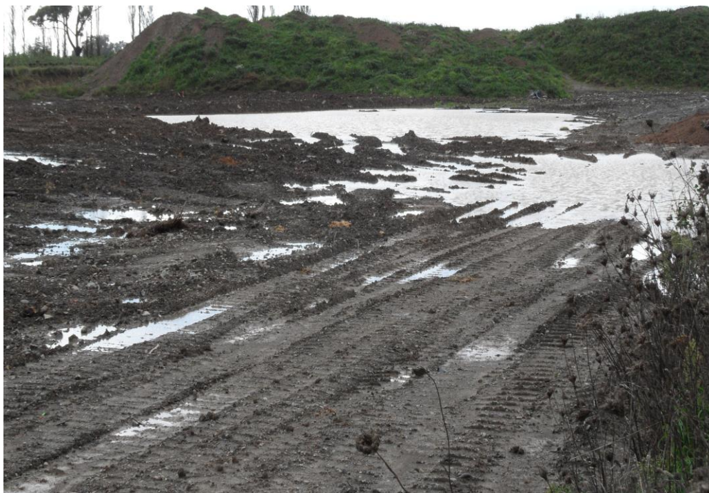
Figure 21. Spreading compaction and drainage impairment.
