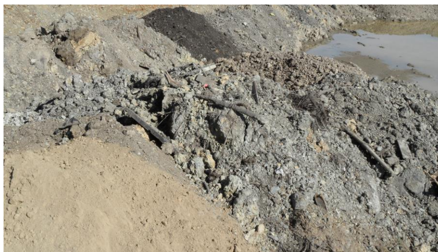
Figure 16. Backfill showing materials being deposited.
