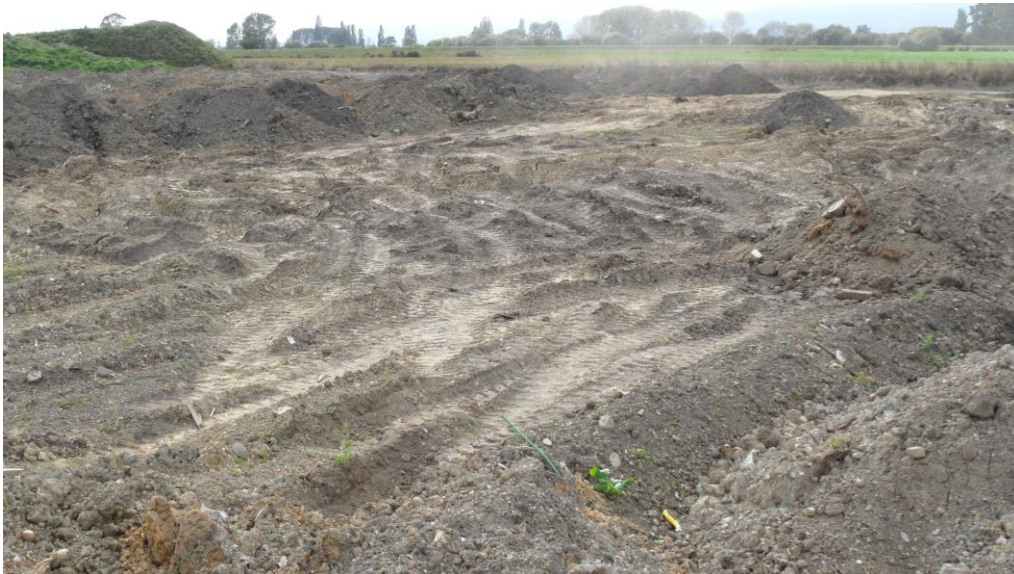
Figure 20. Earth spreading and compaction.
