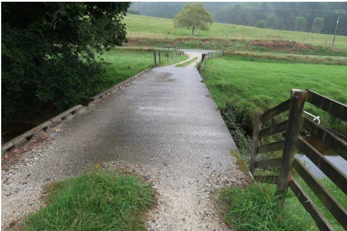
Fig. 3 Bridge over Peach Island overflow channel.
