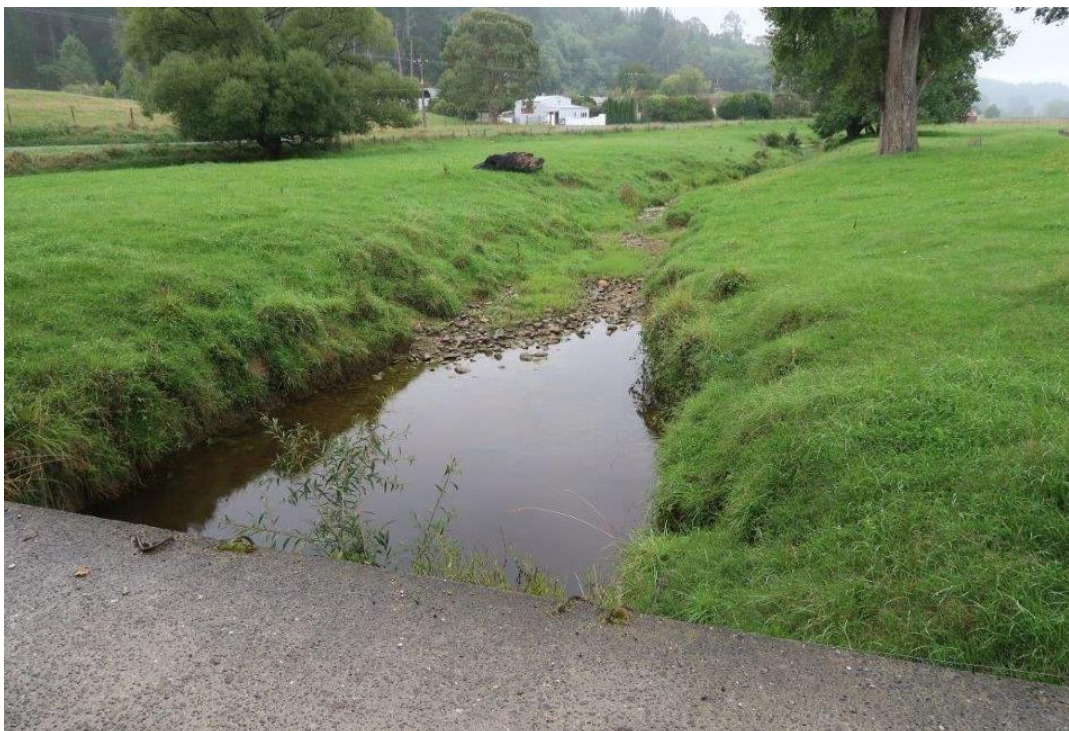
Fig. 4 Peach Island overflow channel immediately downstream of bridge. Dry sections of channel evident.
