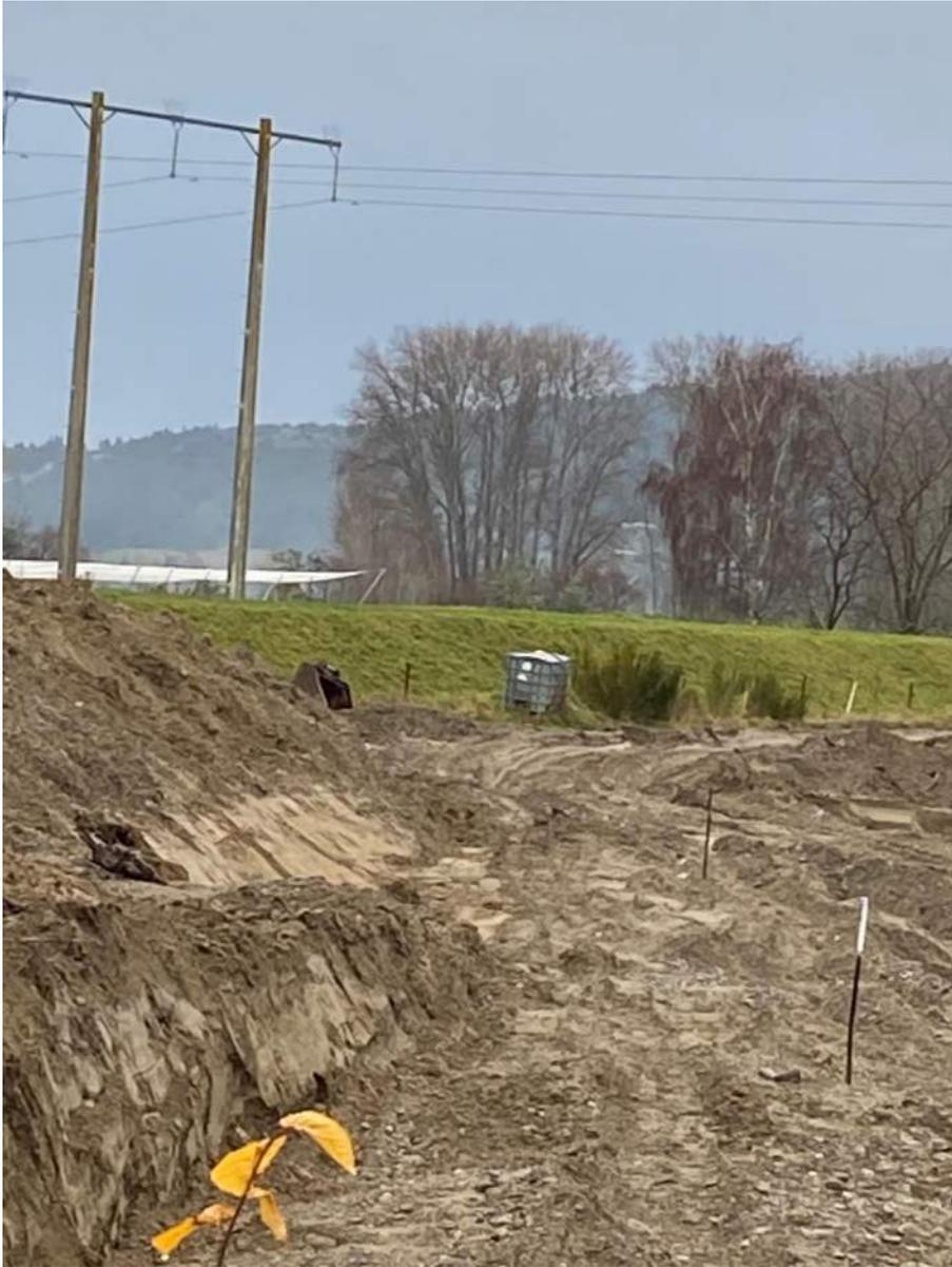
Photo taken on 18 June 22 showing land disturbance and excavation within 20m of stobank toe (shown by markers) and in breach of consent conditions - Dougals Road extraction site. The site flooded two weeks later
