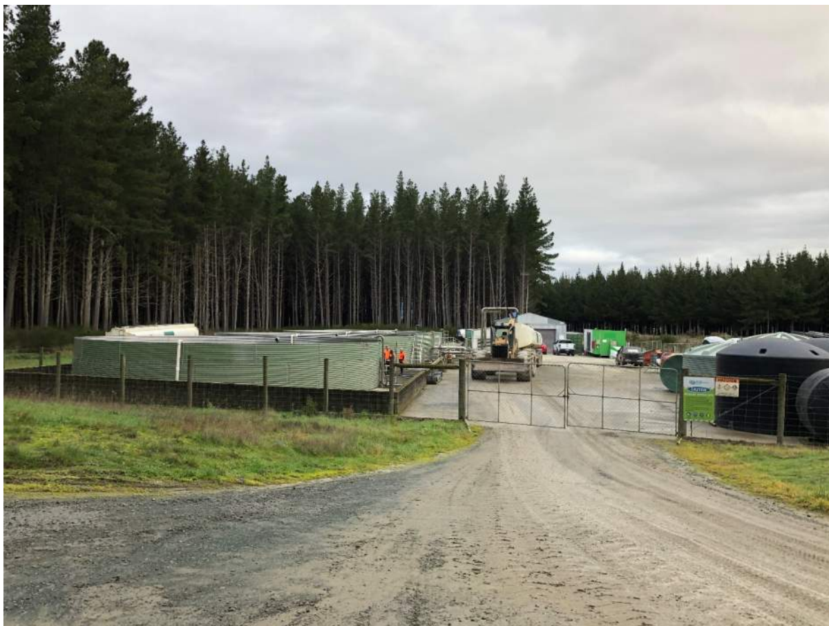
Figure 3: General view of Biosolid Application Facility (BAF)
