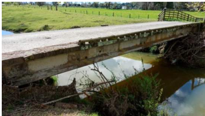
Photo 1: Existing vehicle access bridge
