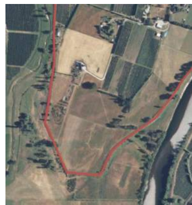
Figure 12: Stop bank location within application site
