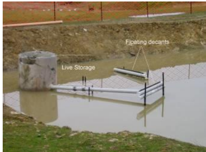
Figure 13-3 Sediment Pond with Floating Decants also Showing Live Storage
