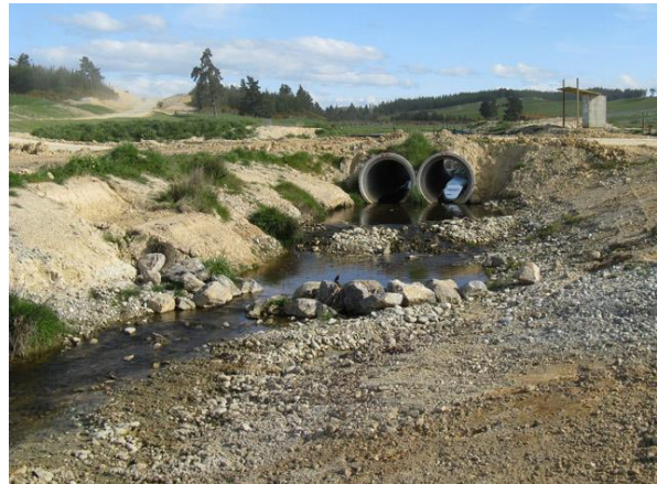
Figure 11-3 Temporary culvert crossing
