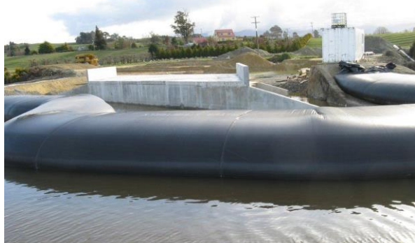
Figure 11-10 Aquadam used on the Ruby Bay bypass to isolate an estuary work site
