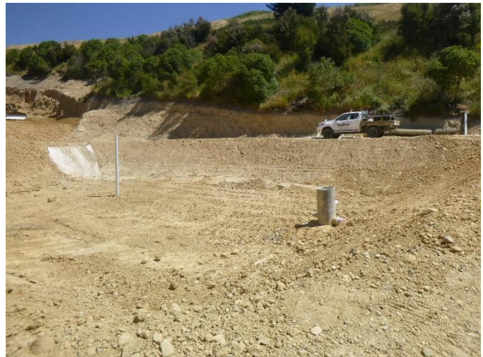
Figure 9-11 Construction of a Sediment Retention Pond
