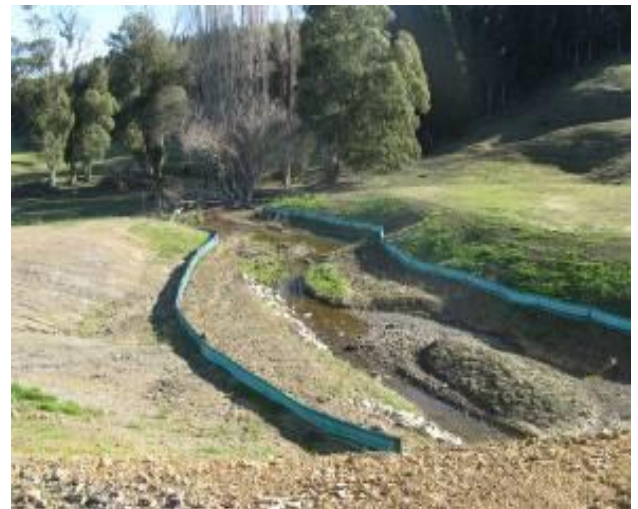
Figure 6-4 Silt Fence Provided for Stream Protection
