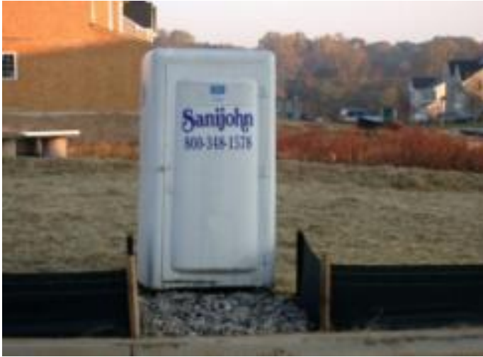
Figure 10-2 Good example of a port-a-loo placed in a location with consideration also given to erosion and sediment controls
