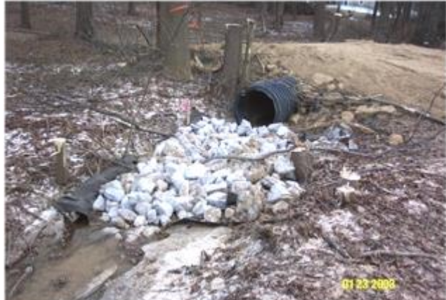
Figure 11-6 Temporary culvert crossing with the rock protection at the outfall to reduce stream erosion
