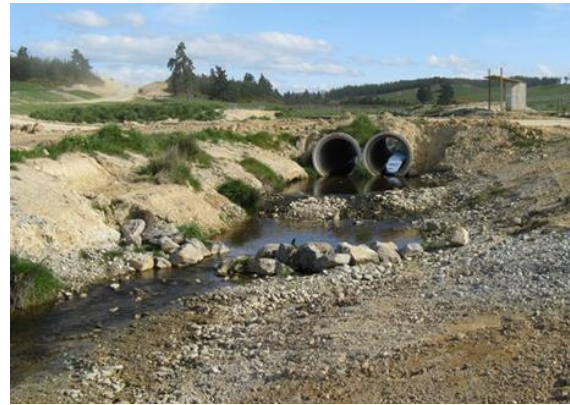
Figure 11-11 Temporary Culvert Crossing
