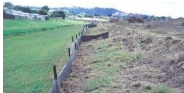
Figure 9-12 Silt fence with returns to reduce lateral water movement
