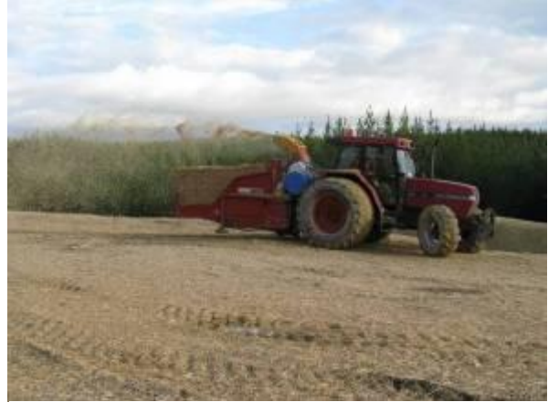
Figure 8-258 Application of straw mulch as a temporary ground cover
