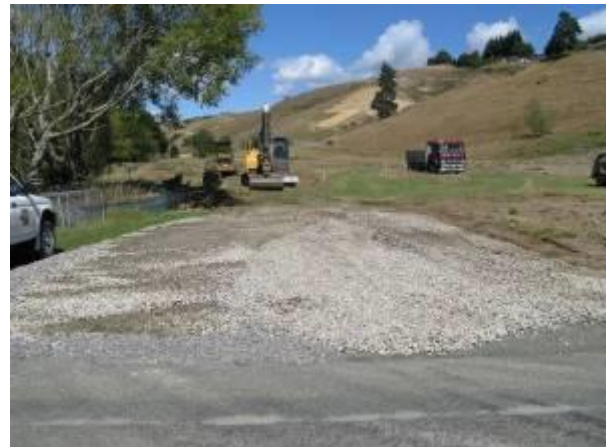
Figure 8-20 Stabilised Entraceways
