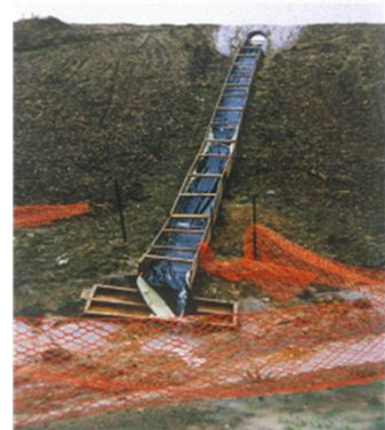
Figure 8-14 Wooden flume lined with impervious material
