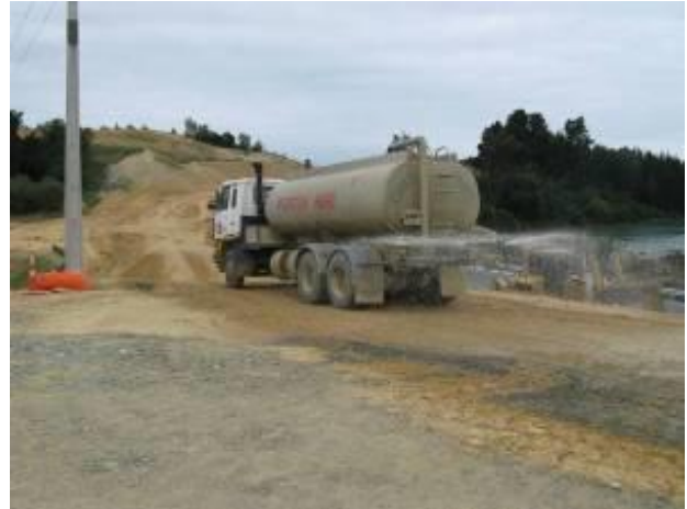
Figure 8-39 Dust suppression by water sprinkling
