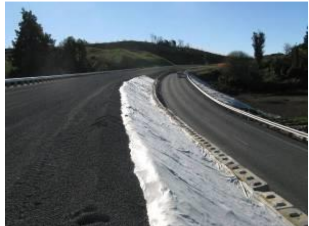
Figure 8-35 Plastic cover to prevent slope erosion
