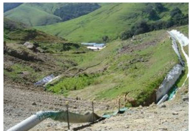
Figure 6-6 Flume Installed to Protect Steep Slope
