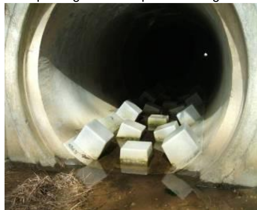
Figure 11-7 Culvert with Energy Dissipation Baffles
