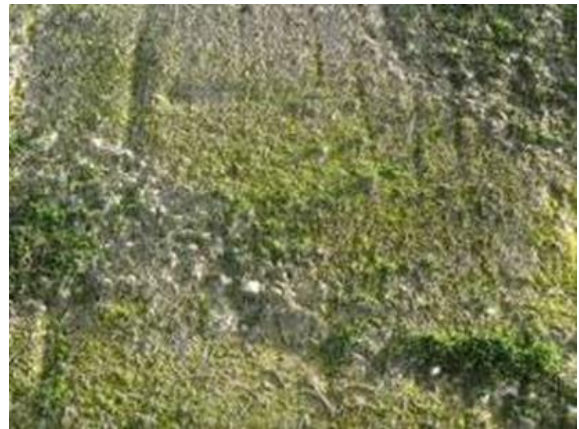
Figure 8-247 Recently applied hydroseed showing emergent grass growth
