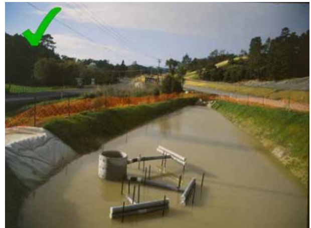
Figure 9-5 Sediment retention pond detail showing multiple decants
