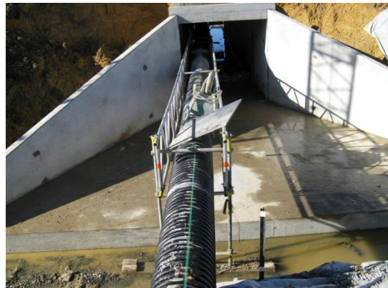
Figure 11-13 Pipe diversion during Ruby Bay Bypass (D.Shaw)
