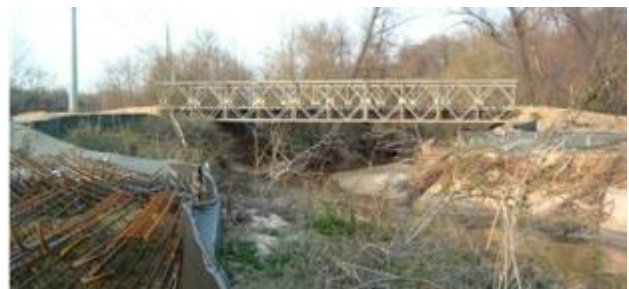
Figure 11-4 Temporary Bridge Crossing
