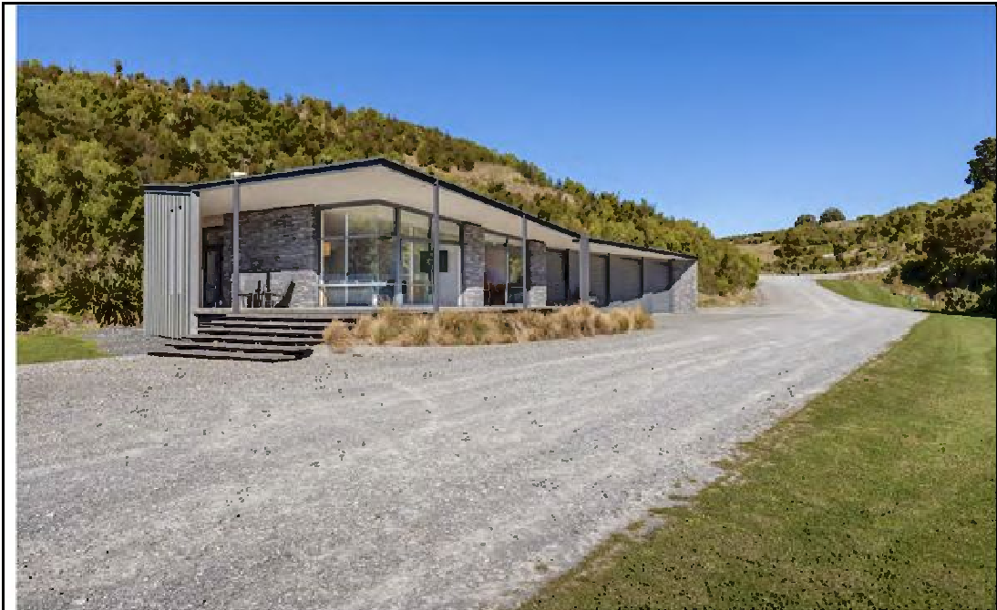
Photo 6: Administration Centre, Machinery Shed & Workshop
