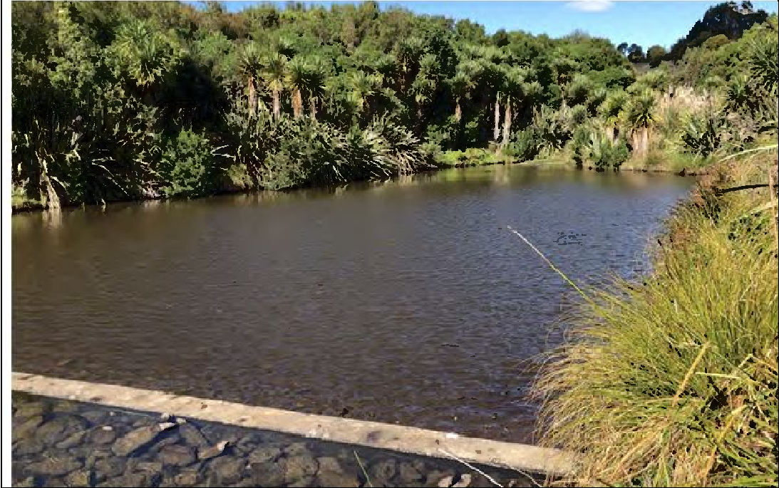
Photo 21: Wetland Bund, Native Plantings and Wetlands
